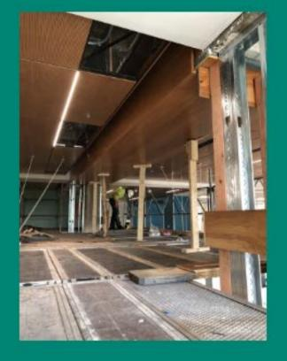
The view from a construction scaffold: wood paneling is installed over a structural beam on the ceiling of the third floor.
